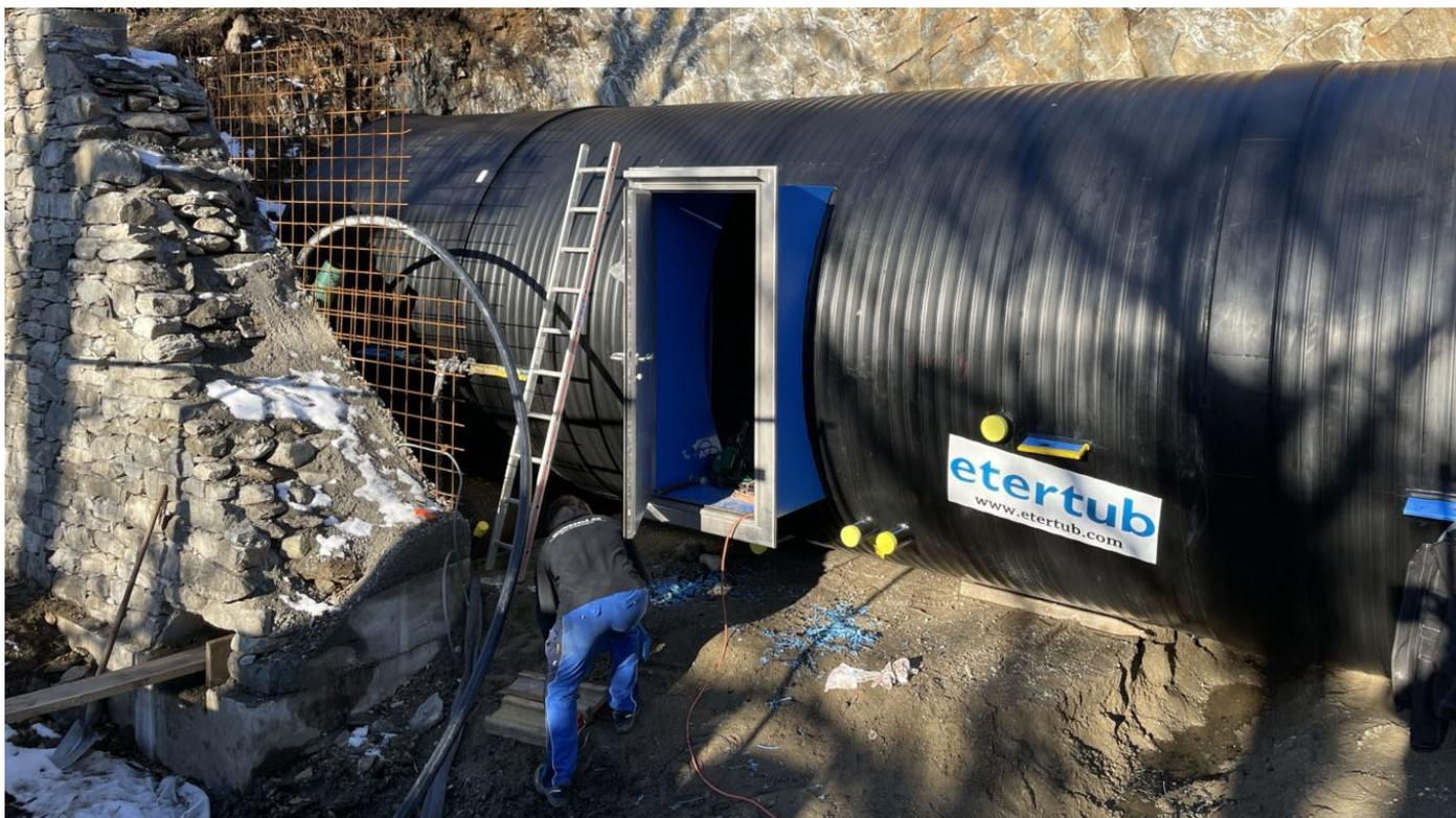
ESEMPIO: CILINDRO SDRAIATO CON PORTA LATERALE D'ACCESSO, IN FASE DI POSA
